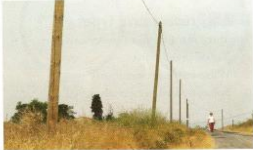
Ⓢ Telegraph poles have to be treated with tar oil preservative to ensure long life
